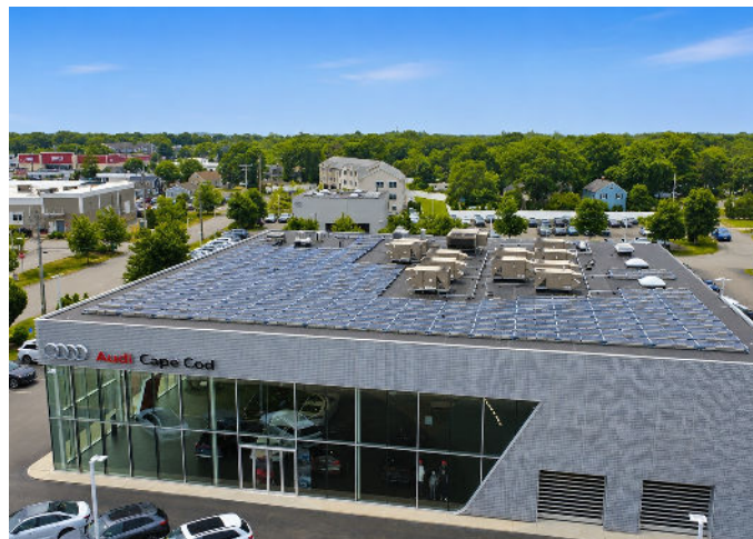
Audi Cape Cod rooftop installation
