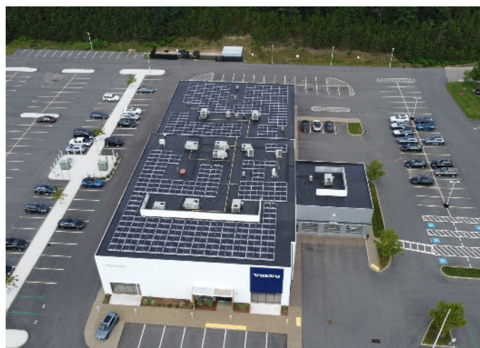
Volvo Plymouth rooftop installation
